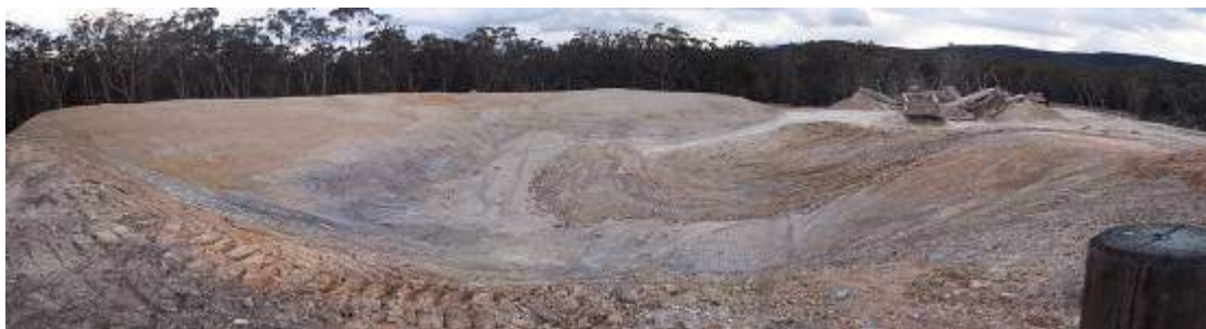
Figure 5 Road base quarry - site 25 revealing deep weathering in chert, soft and hard vein ridden metasandstone and indurated shale. The quarry seems to be in a fault zone associated with the Towrang Fault. Because the quarry has been formed by ripping with bulldozer tines evidence of rock structure has been destroyed.
